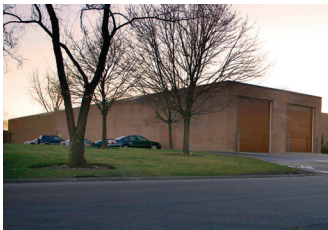
Tool King plant – exterior view
