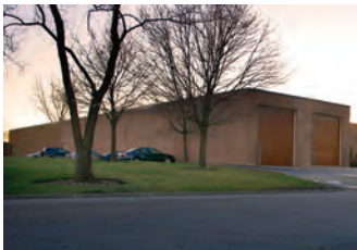
Tool King plant – exterior view
